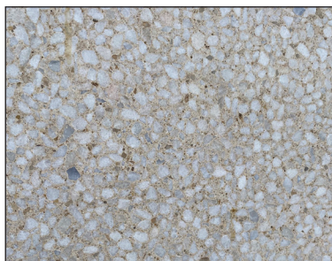
Fig. 16. Polished cement cladding at Locality 15.
