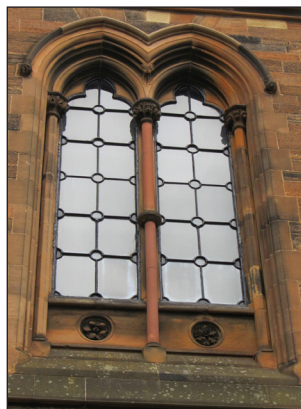
Fig. 7. Window pillars of Old Red Sandstone at Locality 5.
