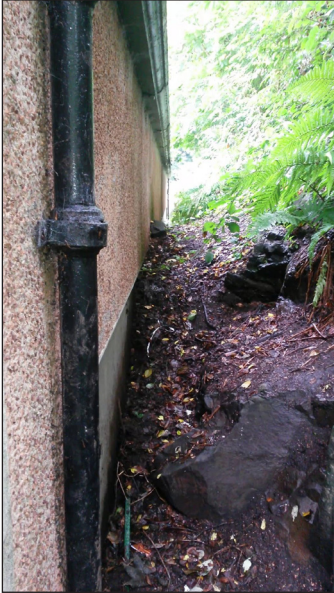
Fig. 1 (Left) Soil and leaf build-up on south elevation. The broken gutter is dripping constantly onto the debris which is saturated. Fig. 2 (above) The tree stump in the lowest position with pooled water and salt efflorescence (arrow). Photo credits D Webster
