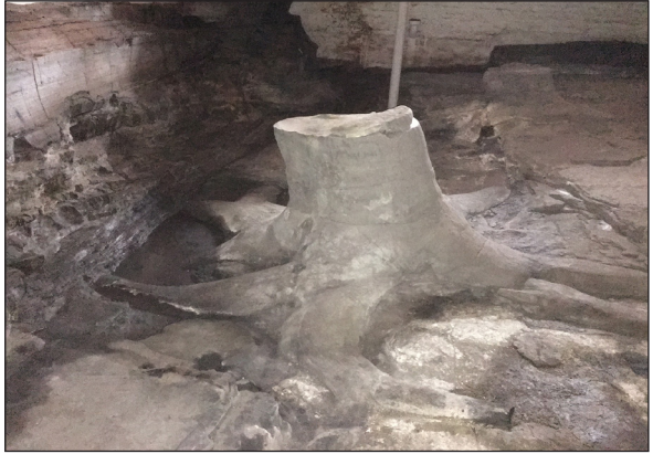
Fig. 1 (Left) Soil and leaf build-up on south elevation. The broken gutter is dripping constantly onto the debris which is saturated. Fig. 2 (above) The tree stump in the lowest position with pooled water and salt efflorescence (arrow). Photo credits D Webster
